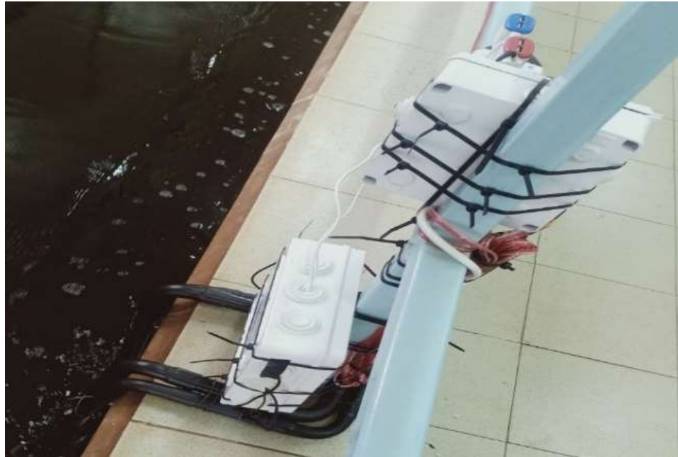
Figure 3.13: A Picture of the sensor node of the WQM System deployed at NYEWASCO
